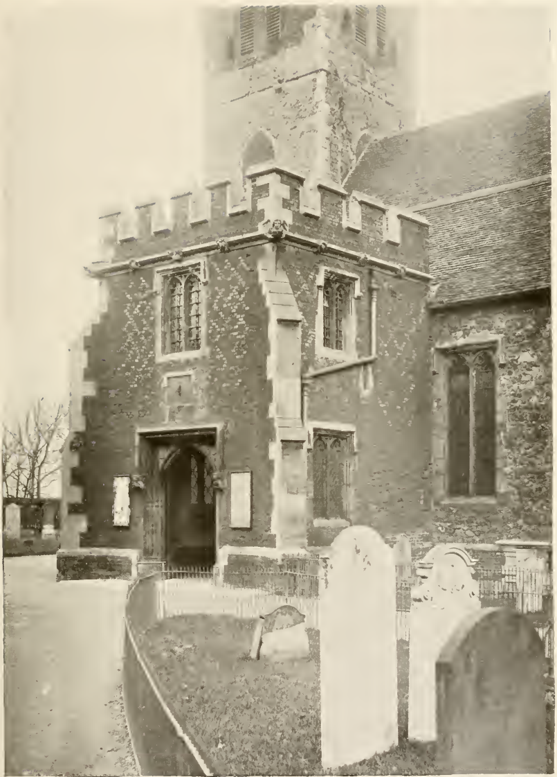
TOTTENHAM CHURCH: SOUTH PORCH.
