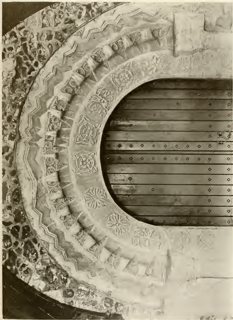
ARCH OF SOUTH DOOR, HARMONDSWORTH CHURCH.
