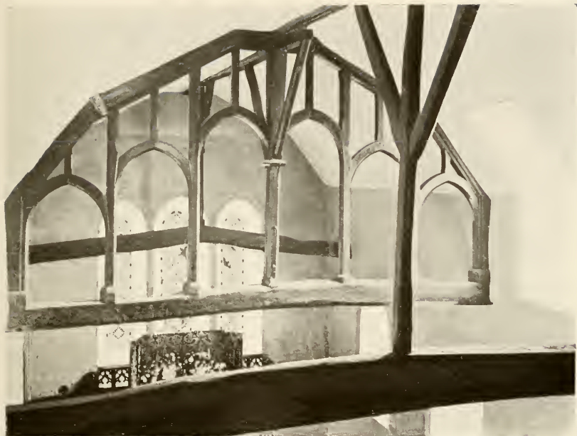
COWLEY : ARCADING IN ROOF-TIMBERS ABOVE SITE OF ROOD-SCREEN.
